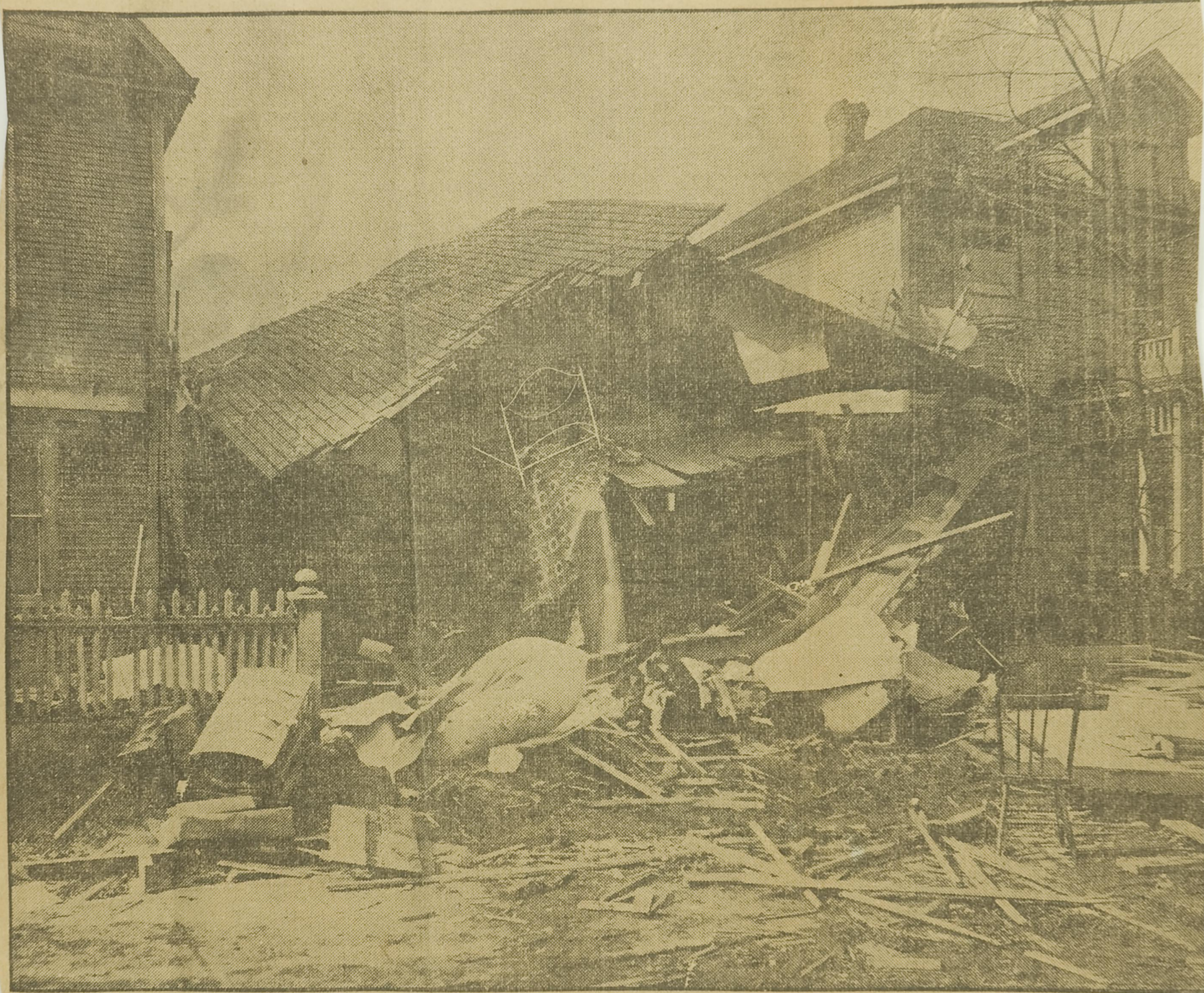
The dynamite bomb which last night exploded in the home of Mutab Sing h, at 1748 Third Avenue west, was placed under the corner of the house directly behind the fence post shown in the picture. A bed in which one Hindu was sleeping is shown in the ruins of the upper storey, while a table which stood in the front room can be seen on the roof at the right corner.
